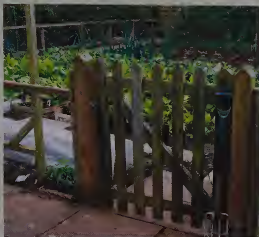
Rabbit-proof fencing should be at least 75cm (30in) high, with 15cm (6in) turned out at the base and buried.
