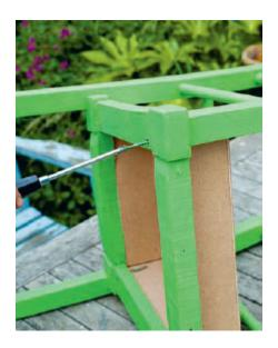
Drill a few holes in the bottom of the chair and then use the screwdriver to screw the wooden box to the underside of the seat.
