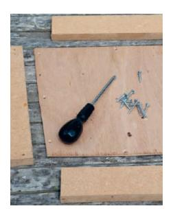
Turn the chair upside down. Measure and cut four pieces of baton to form a box under the seat and a piece of hardboard to form the box base. Ensure the batons for the front and back edges of the box are slightly shorter at both ends (i.e. by the thickness of the batons) so they'll sit neatly between the side batons. Pre-drill three equally spaced holes along the side
