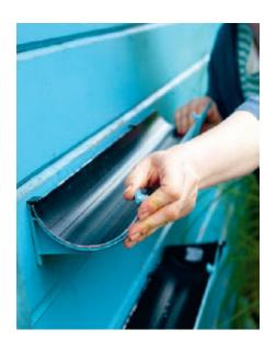
Slide the lengths of guttering onto the brackets, pushing them firmly into place. Re-touch any scratches with some more paint. Fix the end pieces into position, clipping them on securely. Drill a few holes in the bottom of the pieces of guttering for drainage.
