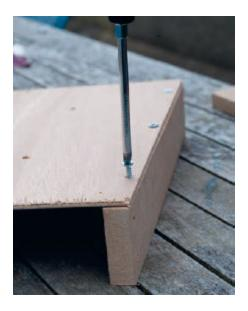
**2** Using the pre-drilled holes, screw the piece of hardboard on top of the batons that will form the sides of the box, using wood screws.
