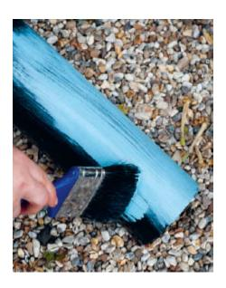
Using the paintbrush, paint the guttering, end pieces, and brackets, leaving the inside of the guttering unpainted. Apply two coats of paint if necessary and leave to dry.
